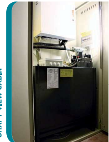
SHAFT VIEW CABIN
